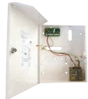
The complete power supply station with 3A switching power supply, PCBA and 2A fuse
